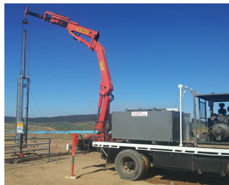
Installation by cargo crane
